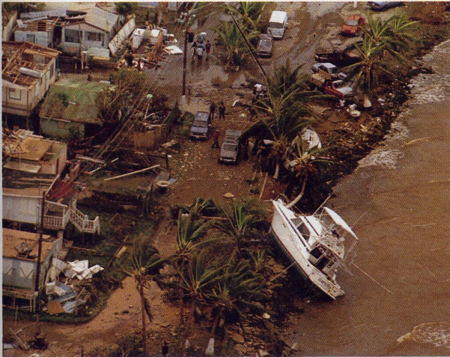
(a) STORM DAMAGE
