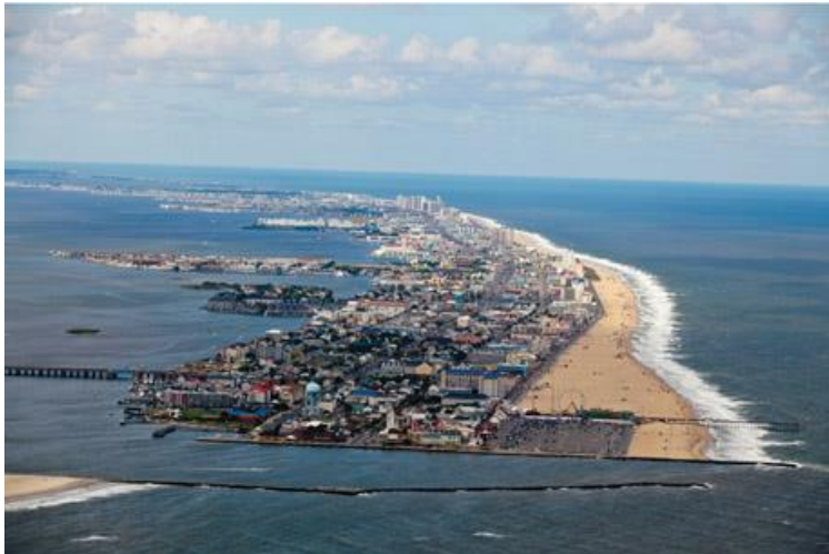
Figure B11.07a: This is an aerial view of Ocean City looking south. The eroding Assateague Island can be seen in the extreme upper right corner of the photo.
